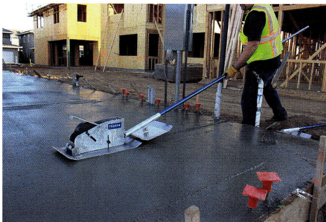
Fig. 5: This manually operated tool is used to embed a polymer tape into fresh concrete. The tape creates a stress concentration in the hardened concrete, typically resulting in a relatively straight crack that opens as the concrete shrinks ( photo courtesy of Aaron Hilbert LLC )
