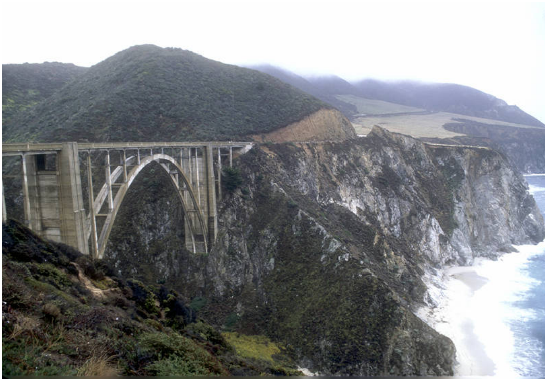
Old concrete arch bridge on California Highway 1
