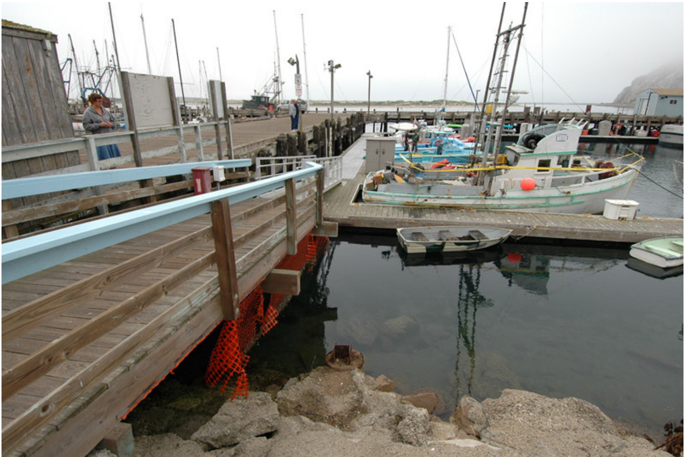
Exit point at foot of pier on northwest side
