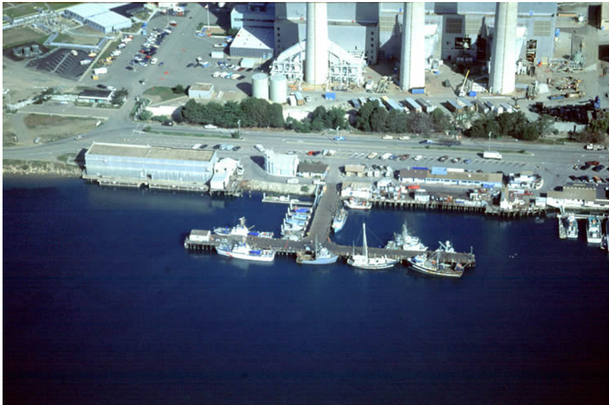
North T-Pier (Coast Guard Pier), Morro Bay, looking northeast
