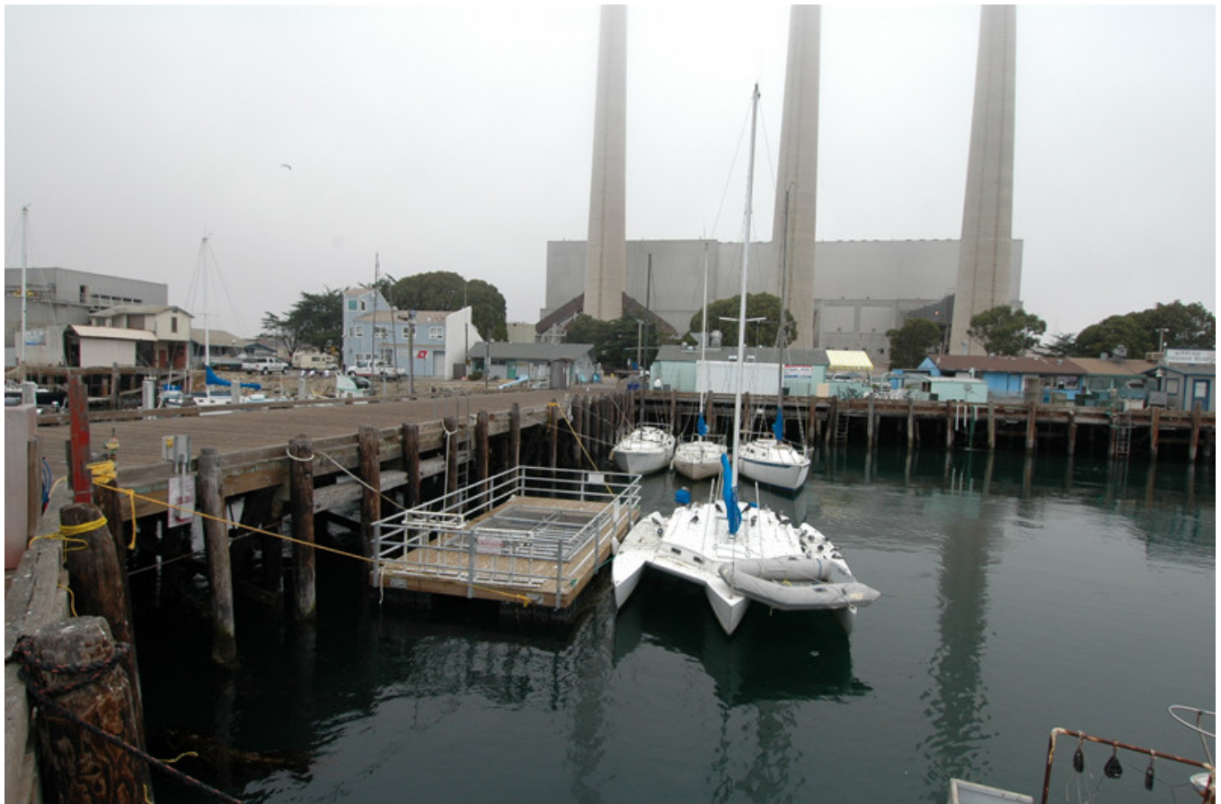
Coast Guard Pier looking north toward stacks, entry point at extreme left where pier bends
