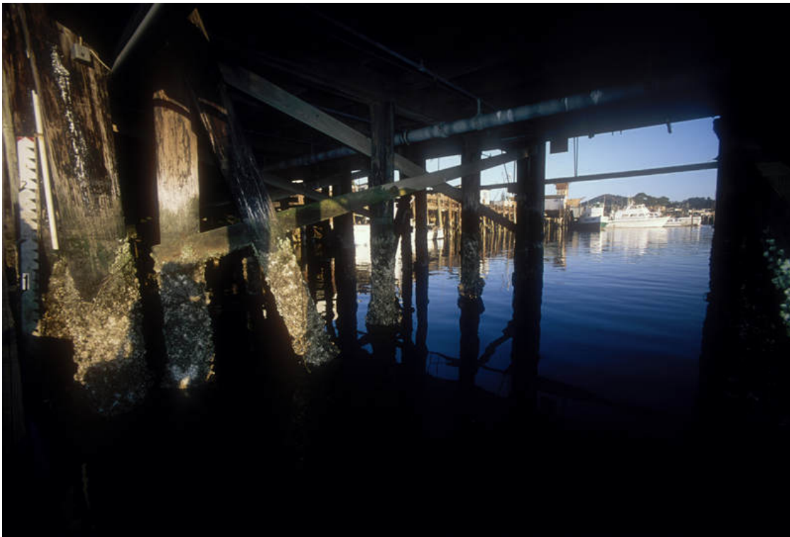
Pier piling and superstructure looking southeast
