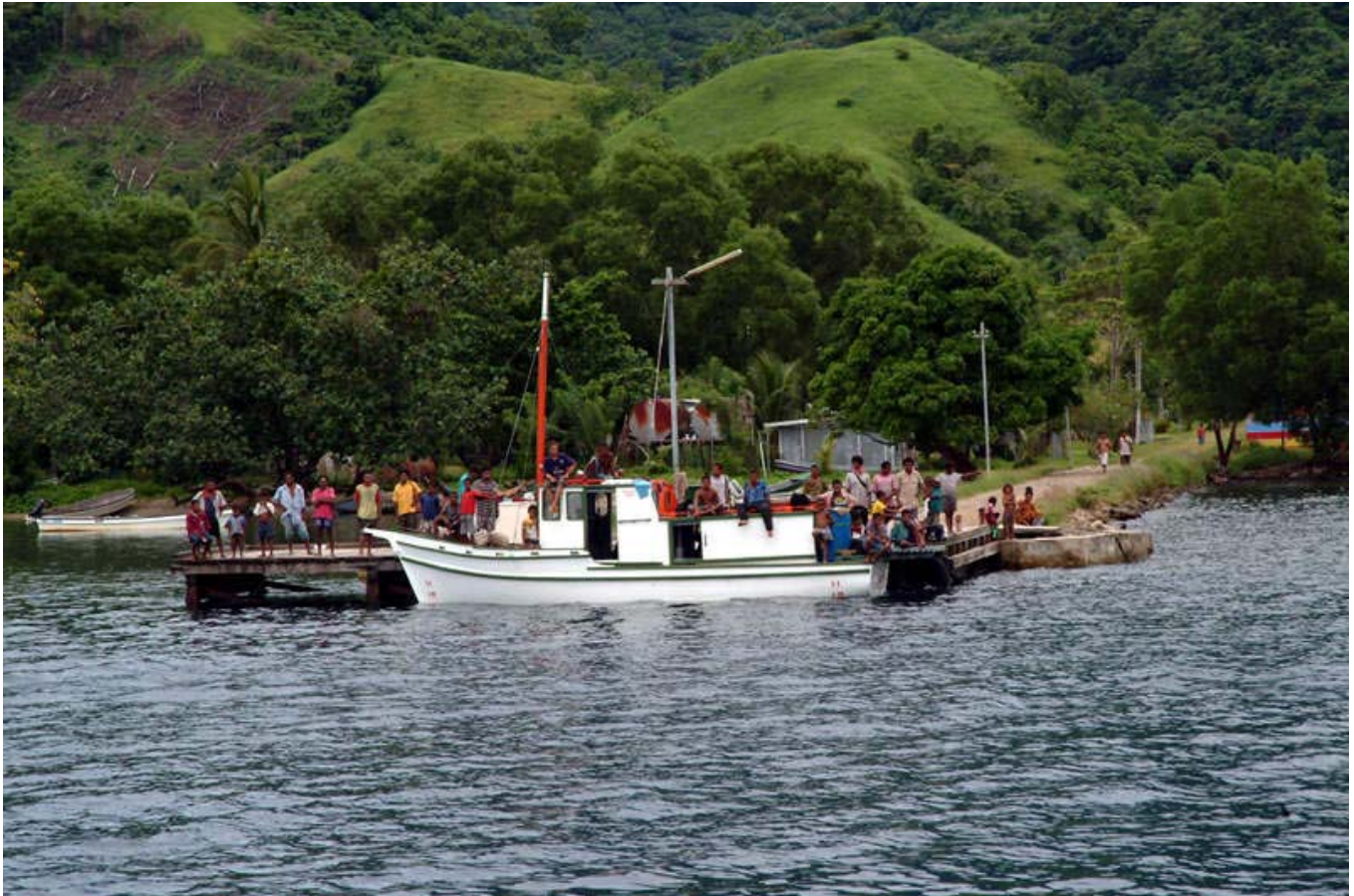
Esa' Ala Wharf above water
