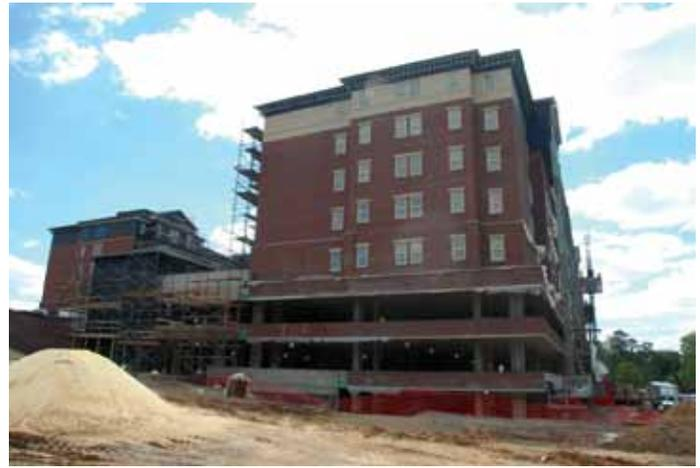
Figure 5: North elevation showing three lower parking levels and five upper residential levels.
