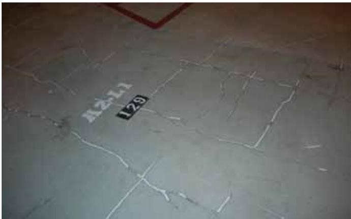
Figure 2: Typical repaired cracks on structure A2 Level L1.
