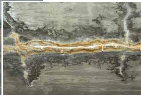
Figure 1: Efflorescence at crack on L1 slab soffit.
