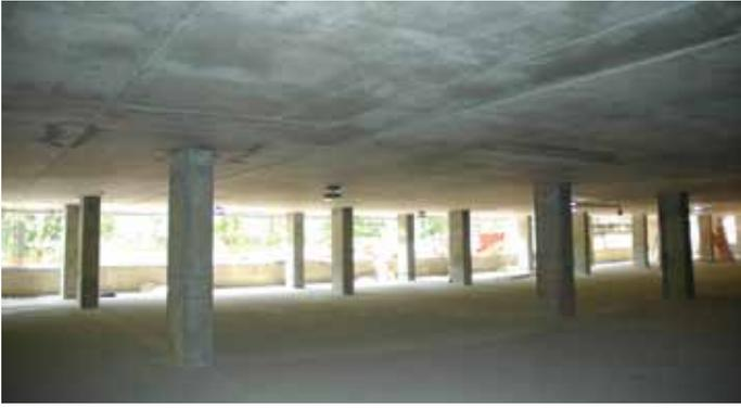
*Soffit of First Level slab (standing on slab-on-ground) looking northwest. The first supported level is the most susceptible to RTS cracking.*
